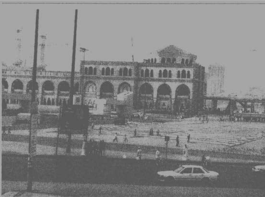
READY FOR PILGRIMS: The extension of the Masaa (a long chamber running between Al-Safa and a few days is expected to increase capacity to 300,000 pilgrims per hour. Over 3,000 construction workers have been working around the clock to complete the SR2.99 billion project. The Masaa is now 20 meters high and includes a newly constructed third floor and a 95-meter-high minaret. (AN photo by Badaa)
